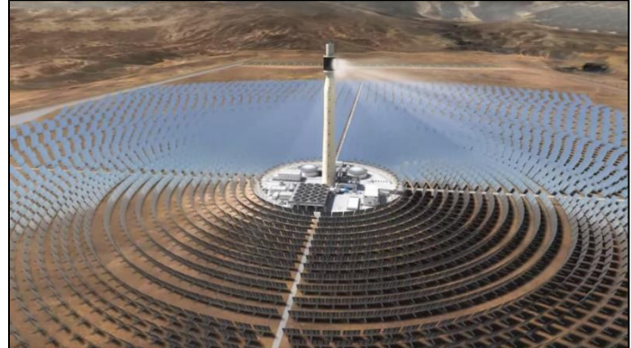
Figure 1. A concentrating solar energy generation field centered around a collection tower holding a central receiver target.
