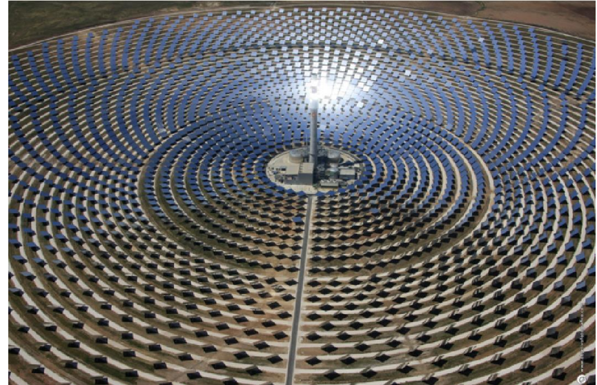
Gemasolar concentrated solar power project Image courtesy of Sener Group
